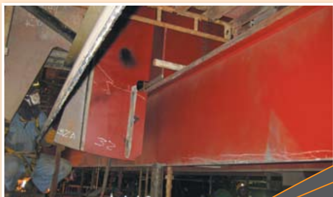
Repairs in progress
