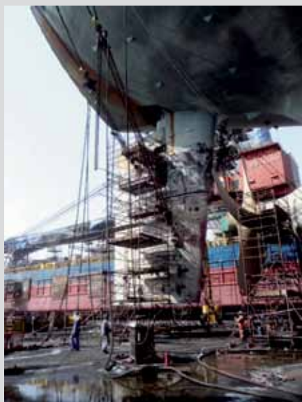
▲ Yard prepares rudder for lowering.
