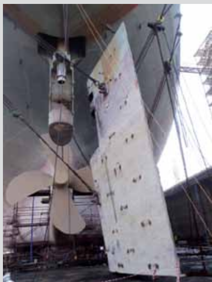
▲ Rudder lowered out
