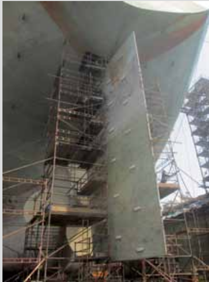
▲ Staging being erected around rudder.
