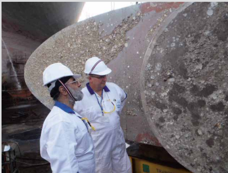
▲ Frontline's Olav Eikrem inspecting bottom pintle on rudder blade with SeaTeam's BK Singh
